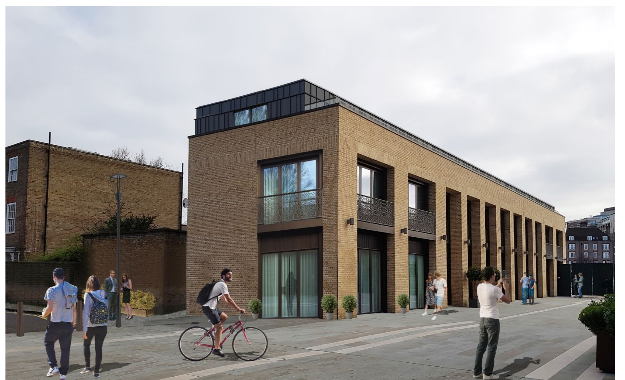
Refurbished Phase 3b containing residential units
