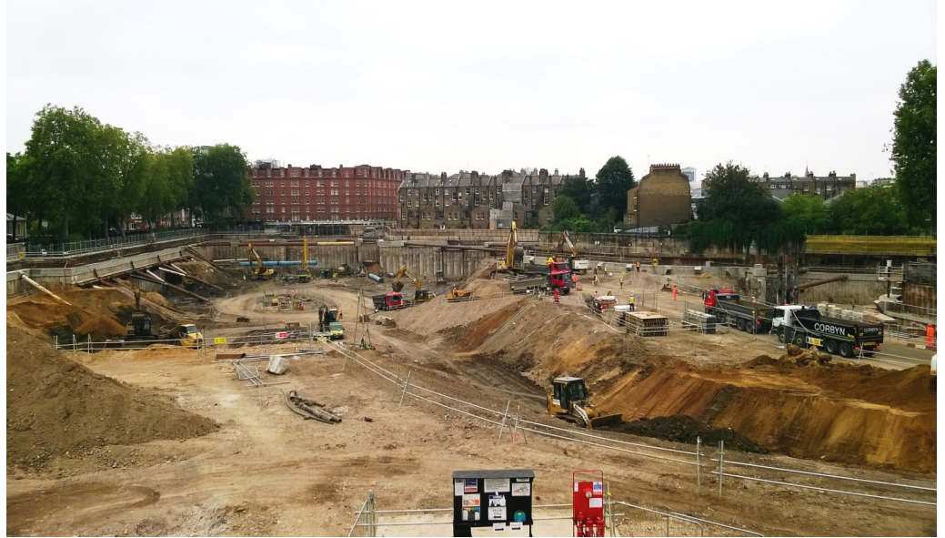
Phase 1 Basement excavation in progress
