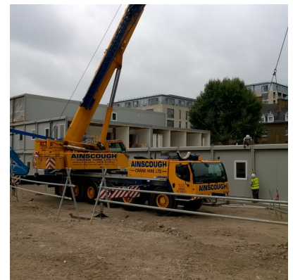
New Site Accommodation being installed
